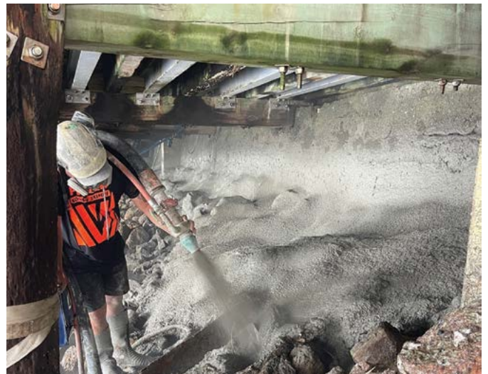
SEA WALL REPAIRS THE STRAND, TAURANGA
